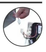
Carefully unscrew and remove the service tunnel and set aside. (This may be required if retrofitting this shower in place of an existing one).
