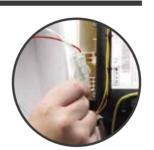
Carefully offer the cover onto the back plate assembly ensuring the wires are not trapped. The control knob, in the fully cold position, may have to be slightly adjusted to enable the key ways
