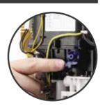
Hold the cover next to the shower unit on the wall and carefully attach the two solenoid connectors. Place the solenoid connector block into the saddle within the shower unit and neatly tuck the wires into the recess provided.
